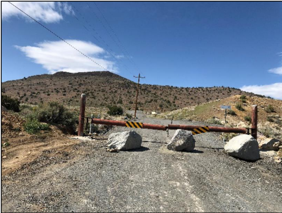
Existing gate across Industrial Parkway, looking north towards the site
