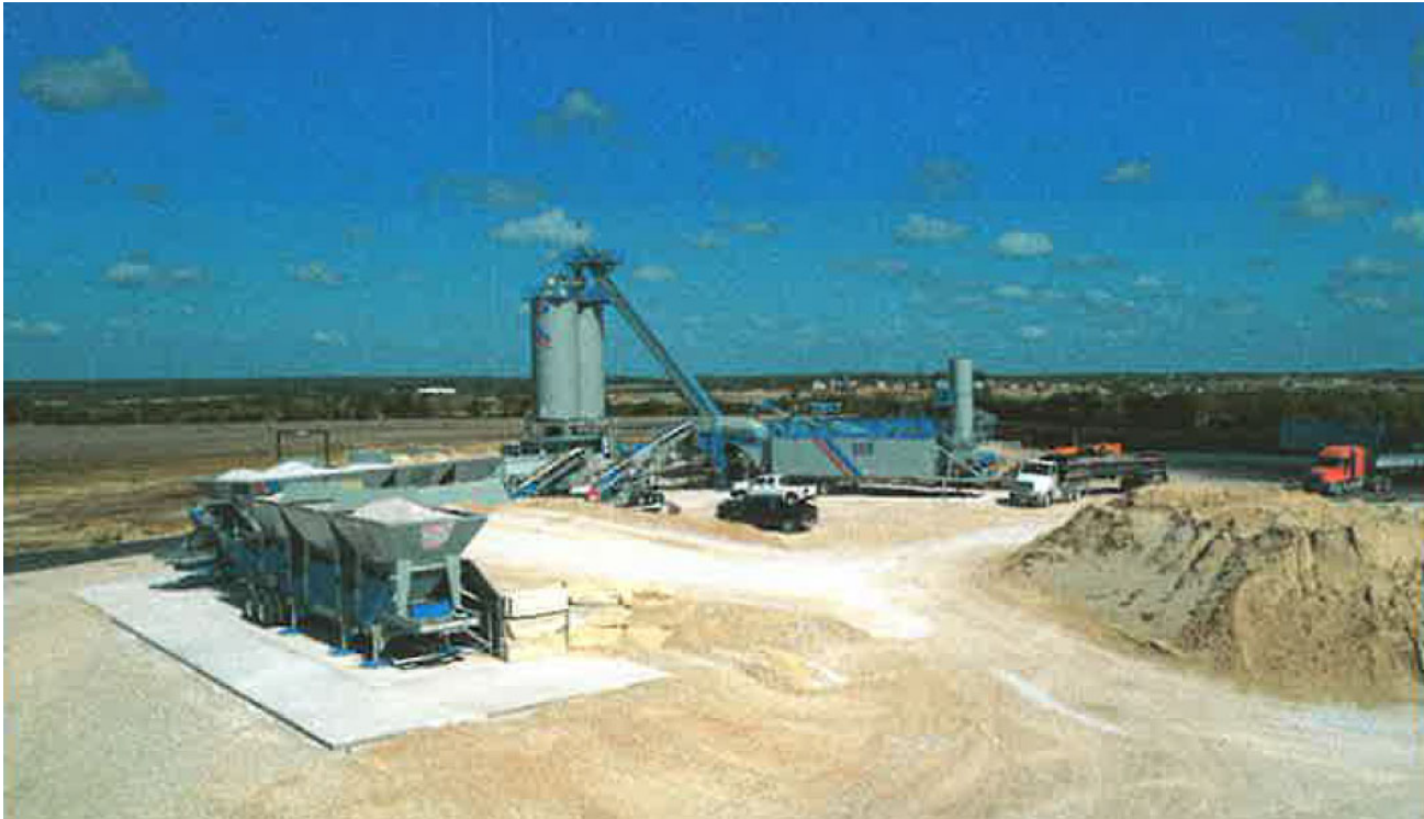
Figure 3 – Example of an Asphalt Batch Plant operation
